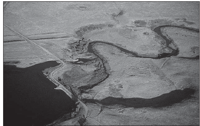
Figure 1. Small earth fill dam – photo courtesy of PFRA
